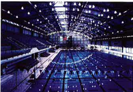
Nassau County Aquatic Center, East Meadow, NY
